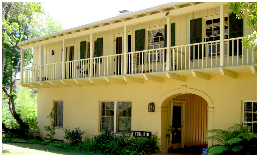
Multi-family Building with second-story protruding Monterey balcony.
