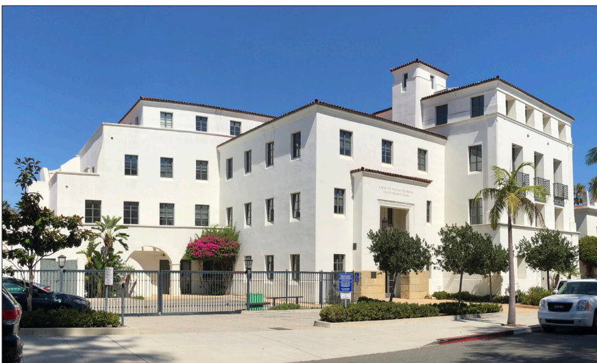
Building designed with two-, three-, and four-story building massing (height averaging).
