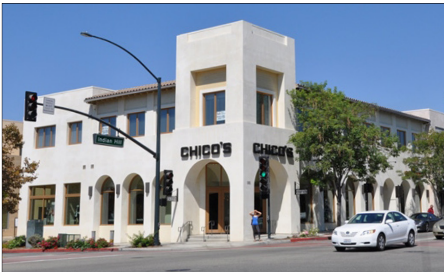
Mixed-use building articulated with corner tower.
