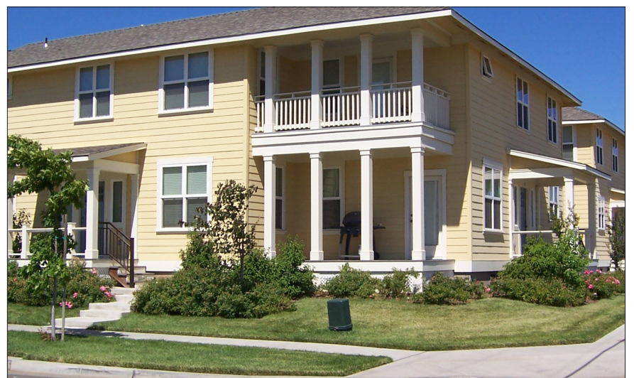
Multi-family building with recessed, double-story balcony (architectural recession).
