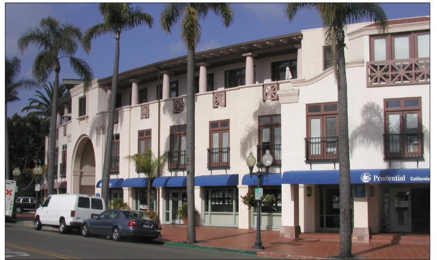
Mixed-use building with recessed third floor balcony and creative differentiation of floors (floor level articulation).
