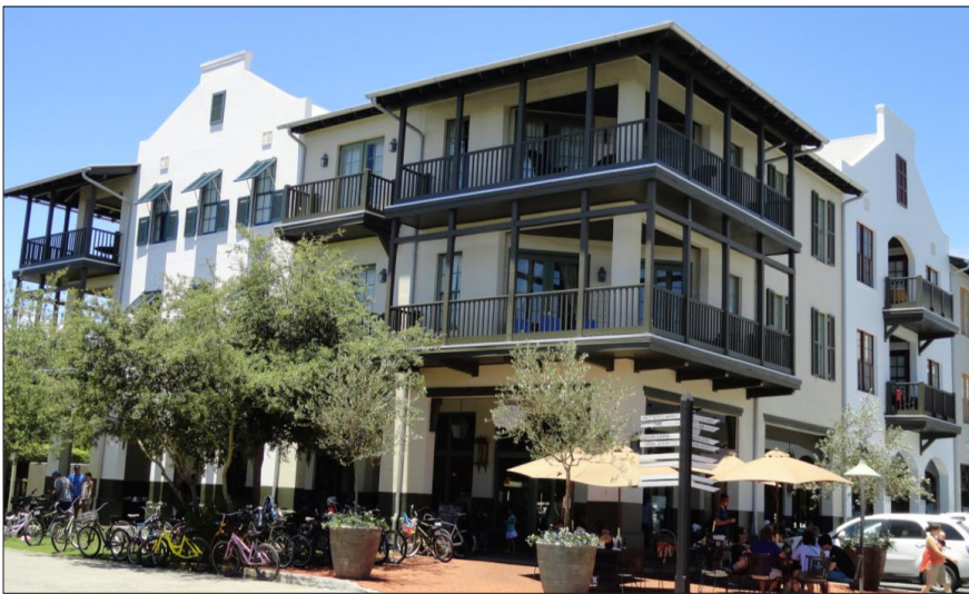
Mixed-use building with protruding Monterey and standard balconies.
