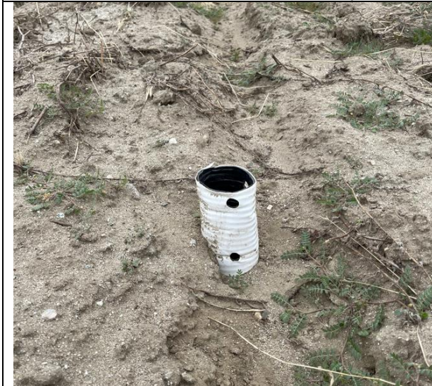
Photo 9. Pipe with drain holes observed onsite.
