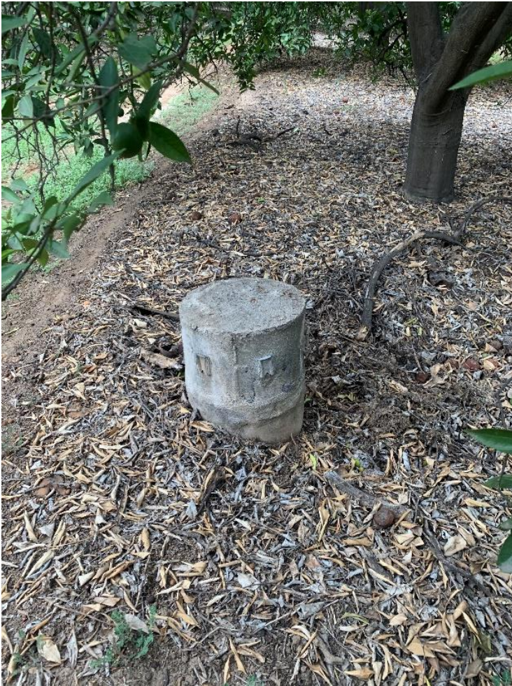
Photograph 5: Detail, a shortened standpipe used for irrigation purposes and located throughout the subject property's orange groves, July 25, 2019.
