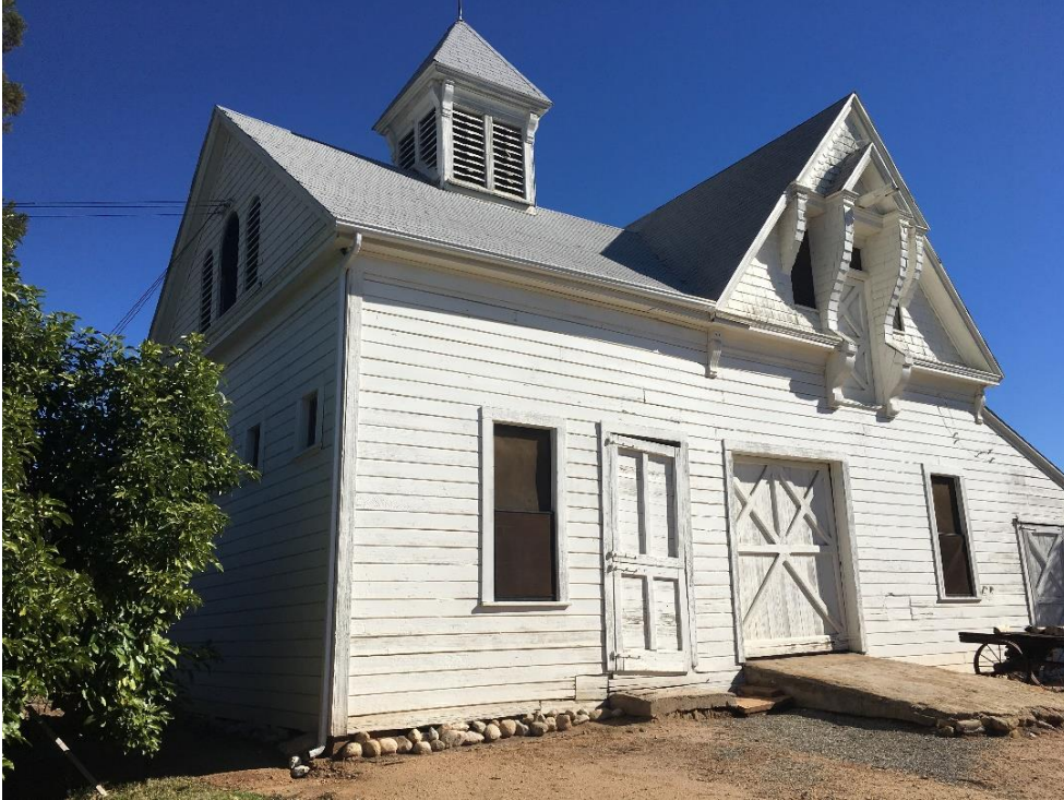
Photograph 11: Northwest and southwest elevations and cement entryway leading to large sliding wooden door serving as structure's main entrance, camera facing east, January 9, 2019.
