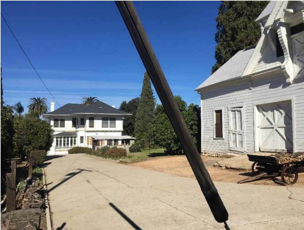
Photograph 2: Southwest elevation of carriage house with southeast elevation of main Palm Avenue residence in background and driveway connecting the two, January 9, 2019.
