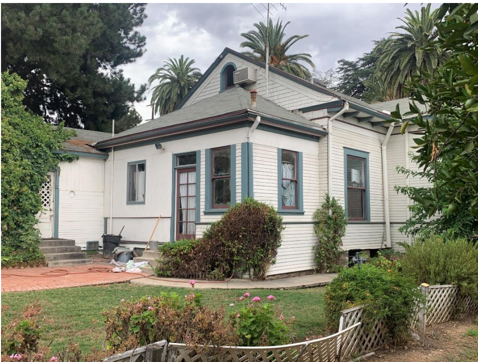
Photograph 11: Northeast and northwest elevations with enclosed back patio also in view, camera facing south, July 25, 2019.
