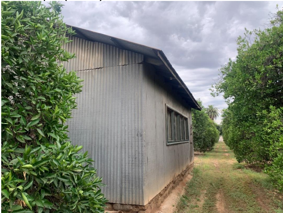
Photograph 2: Northwest elevation of the garage with the northeast elevation majorly obscured by overgrown bushes, camera facing west, July 25, 2019.
