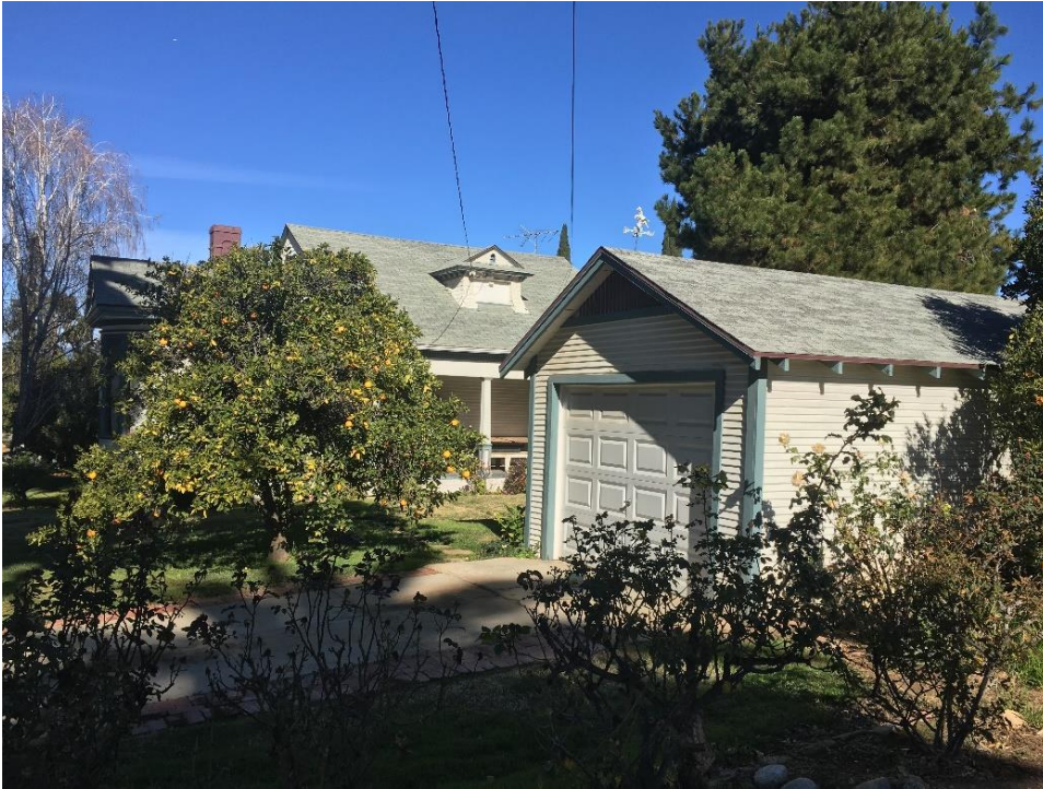
Photograph 12: Alvarado Street residence with detached garage in foreground, featuring a paved driveway and weathervane, southwest elevation, camera facing north, January 9, 2019.
