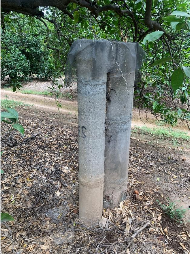
Photograph 6: Detail, two larger standpipes used for orange grove irrigation and watering with the tops covered by mesh screens, July
