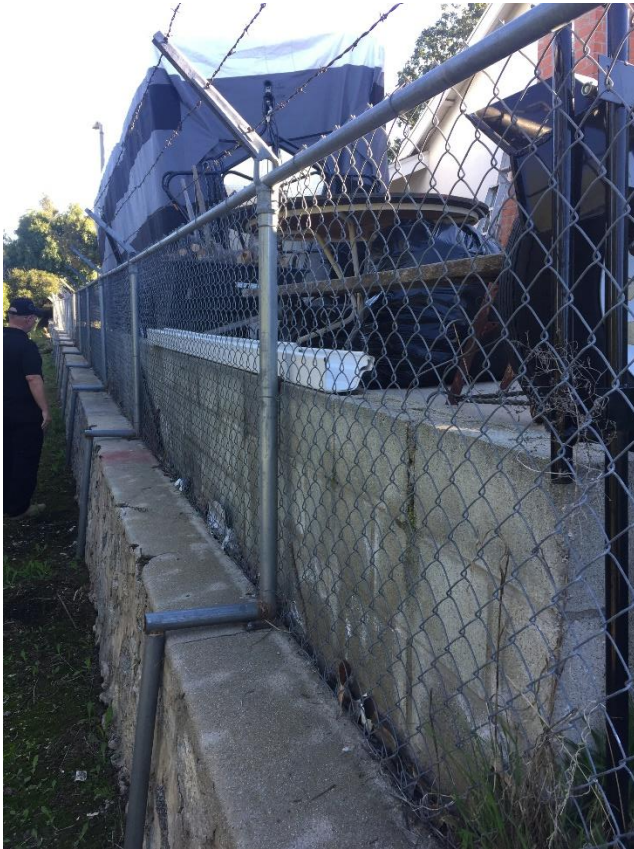
Photograph 4: View of the footing along the southeast property boundary separating it from a neighboring residence, camera facing northeast, January 28, 2020.
