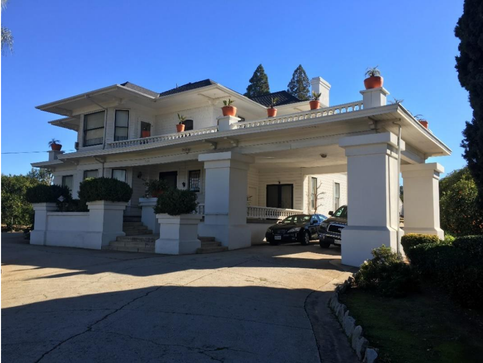
Photograph 2: View of the northwest elevation of the residence and carport from the west side of the semi-circular front driveway, camera facing east, January 9, 2019.
