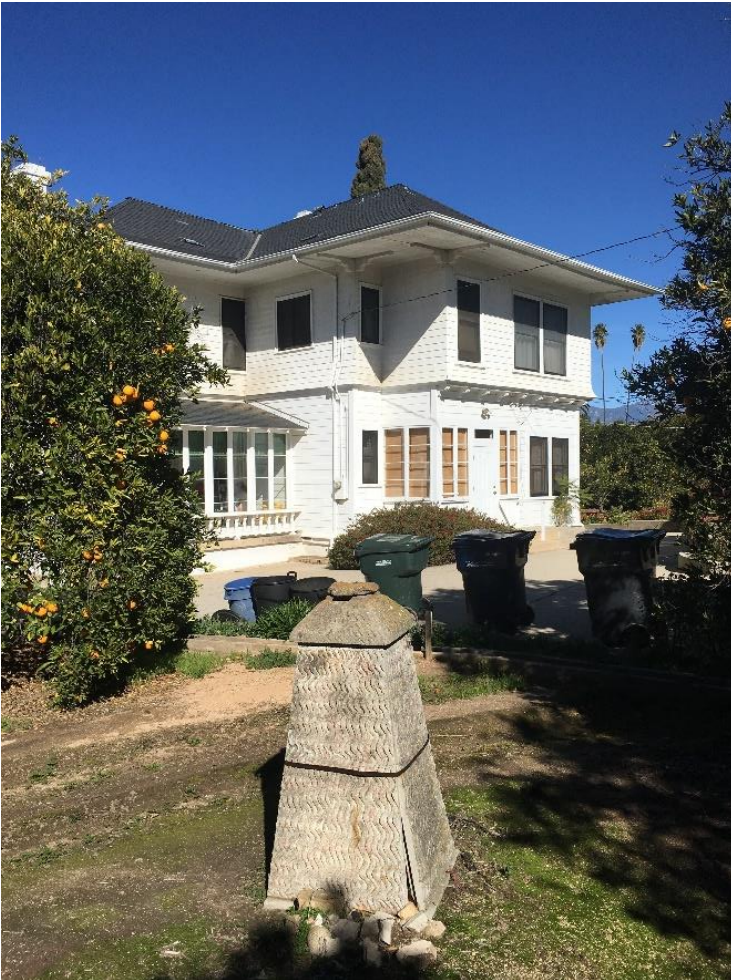
Photograph 10: Detail, incinerator in context of the residence located to the immediate northeast, January 9, 2019.
