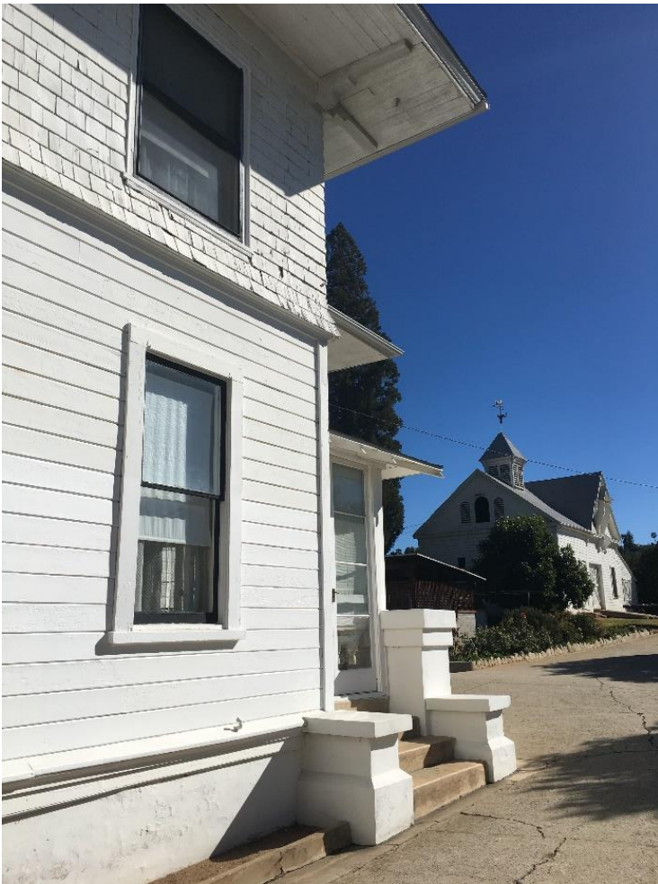
Photograph 6: Detail, wooden siding and backdoor entrance in the southwestern corner of the residence with carriage house visible in background, January 9, 2019.
