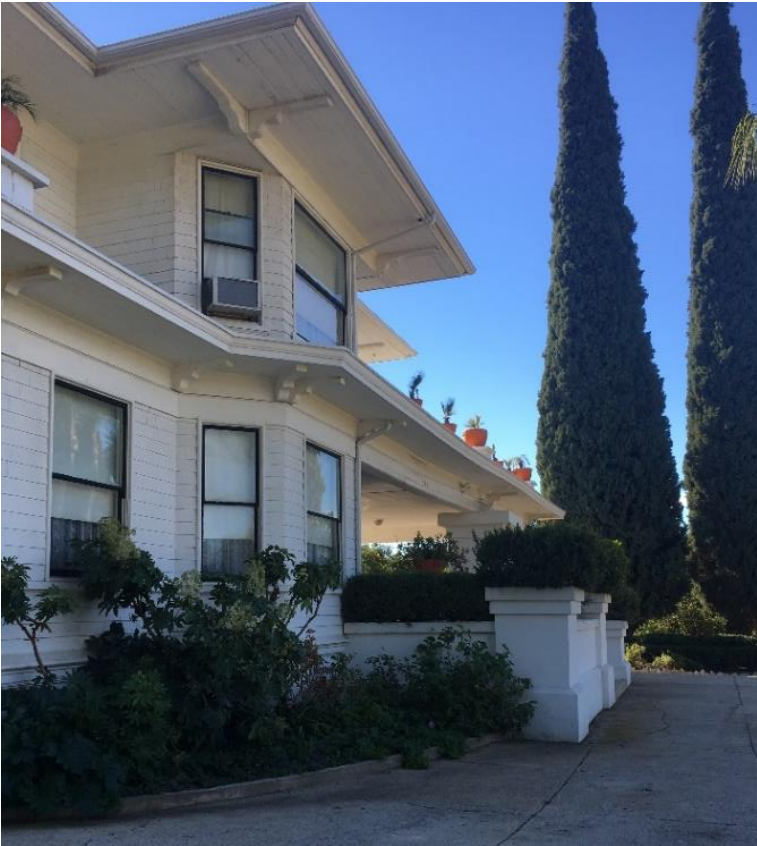
Photograph 4: Detail, frontal windows facing Palm Avenue and eaves, camera facing west, January 9, 2019.
