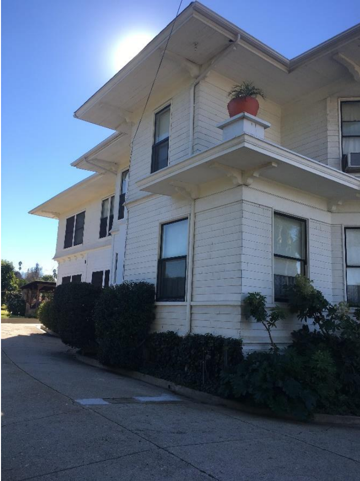
Photograph 5: Detail, windows and siding along the northeastern elevation of the residence, camera facing south, January 9, 2019.
