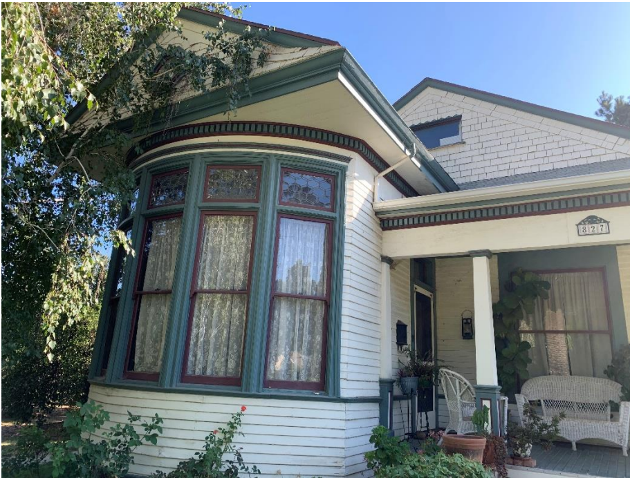
Photograph 4: Detail, front-facing bay windows with ornate glass and painted wooden framing, roofline obstructed from view by trees, August 22, 2019.
