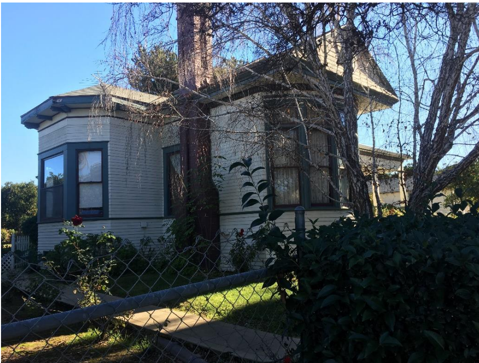
Photograph 3: Alternate view of the front of residence taken from behind fence enclosing the property, southwest elevation, camera facing east, January 9, 2019.
