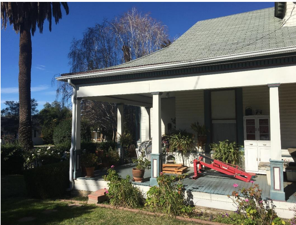
Photograph 9: Detail, close-up of front porch with sloped roof and ornate beam pillars, southeast elevation, January 9, 2019.
