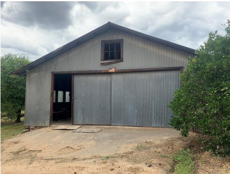
Photograph 5: Southwest elevation, wooden-framed sliding door and windows easily visible, camera facing northeast, July 25, 2019.
