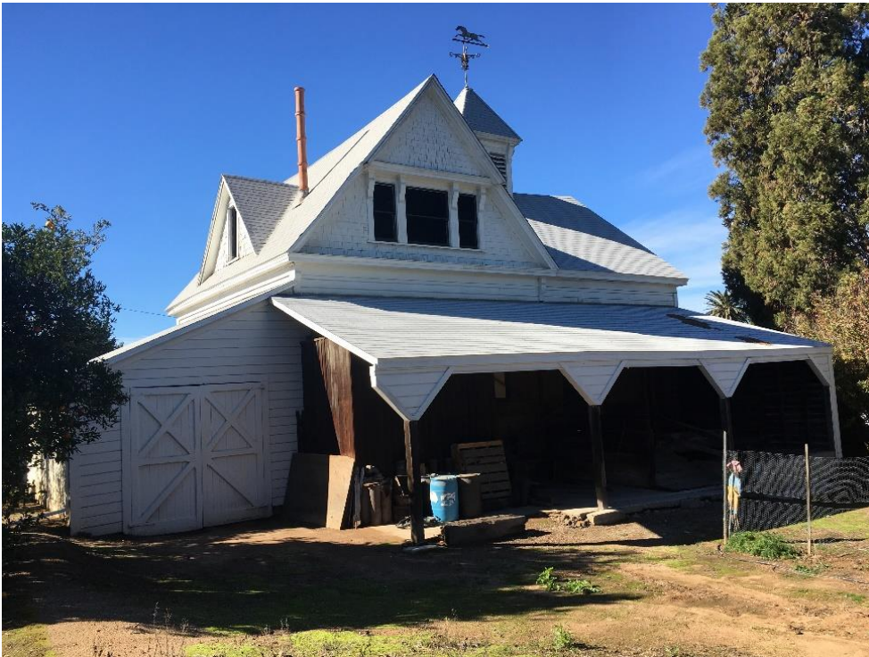
Photograph 4: Northeastern elevation with covered back patio area, camera facing west, January 9, 2019.
