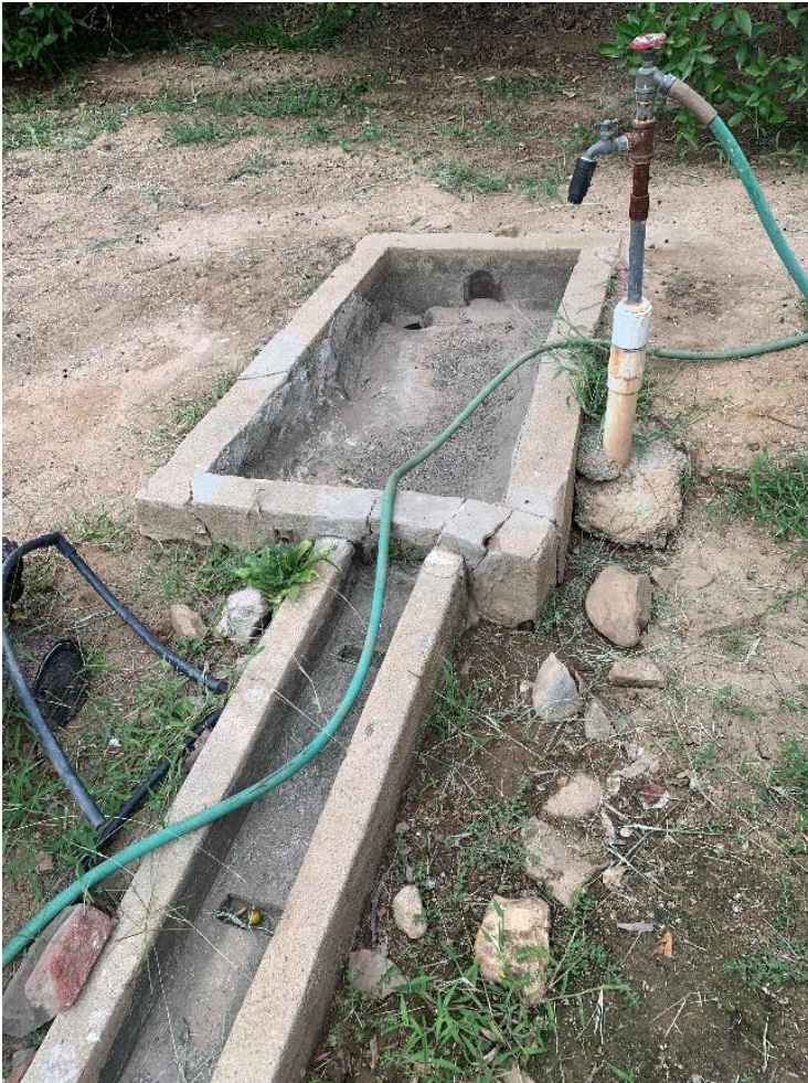
Photograph 3: Detail, gravity-fed irrigation canal connected to a small cement basin at its southeast terminus, July 25, 2019.
