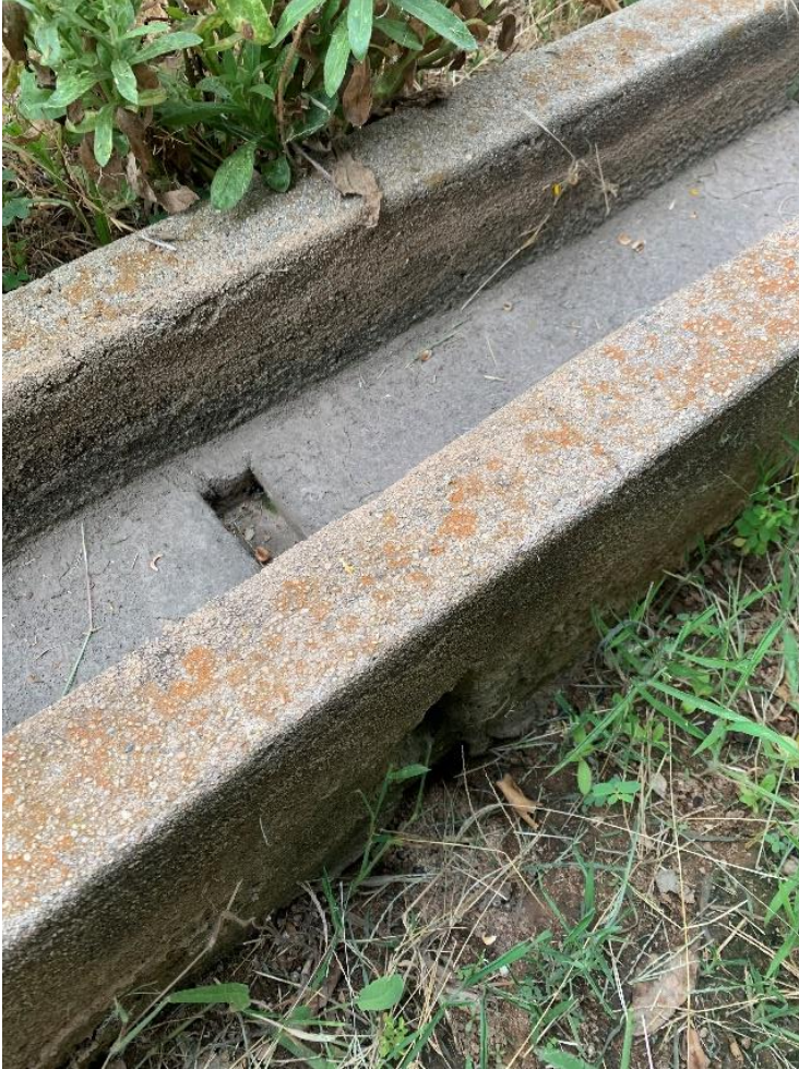
Photograph 2: Detail, cement canal with close-up of the outlet divot, July 25, 2019.
