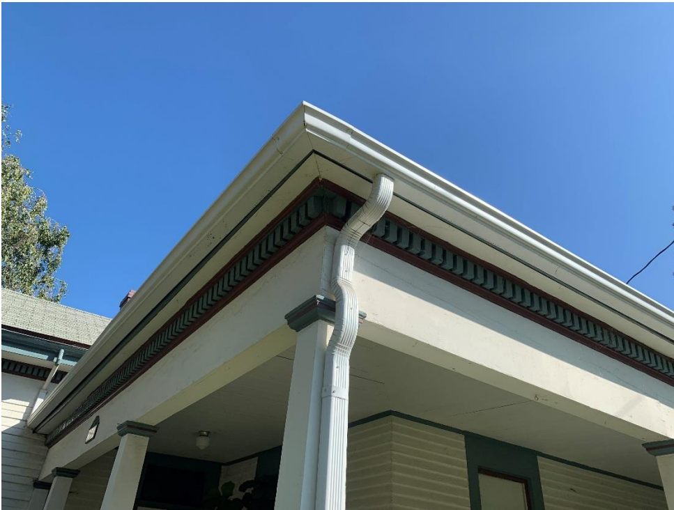
Photograph 8: Detail, decorative painted woodwork ornamentation lining gabled roof, August 22, 2019.
