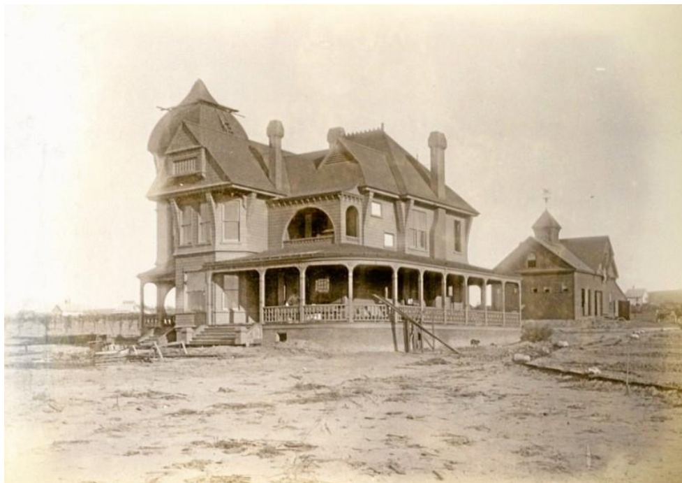
Figure 4: The original primary England residence and carriage house nearing completion of construction, 1891.
