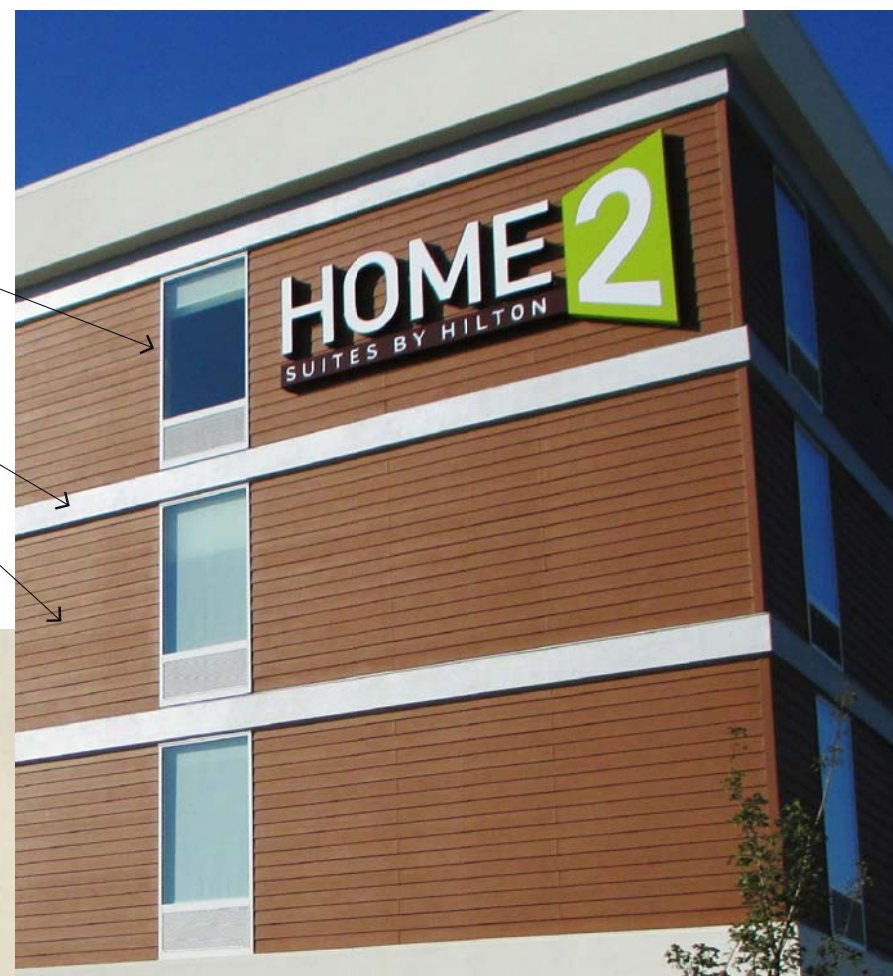
FLUSH FIBER CEMENT SIDING DETAILS
