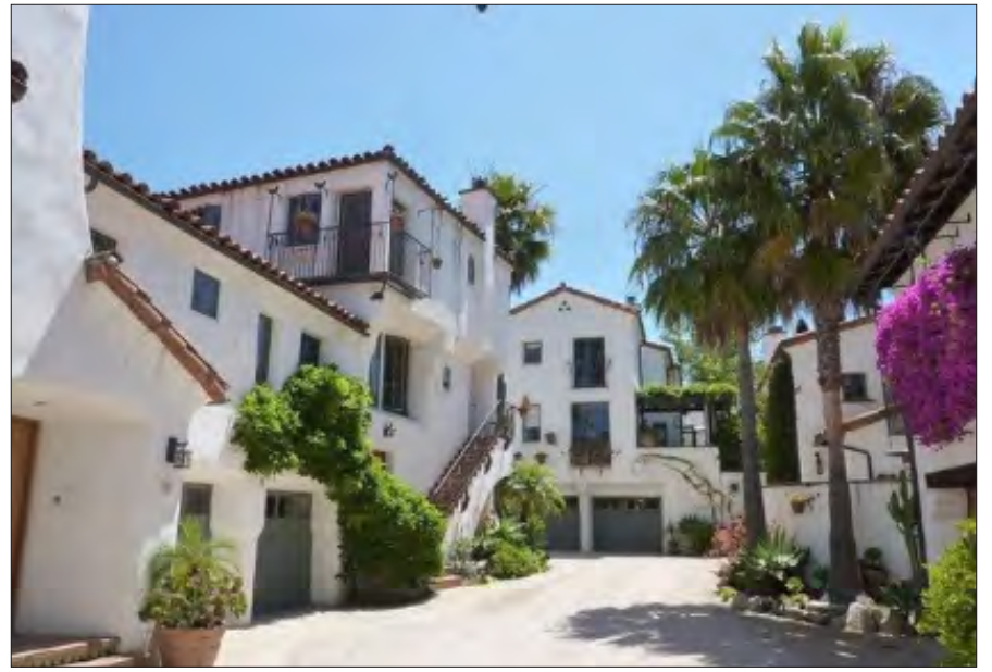
Alley behind multi-family building.
