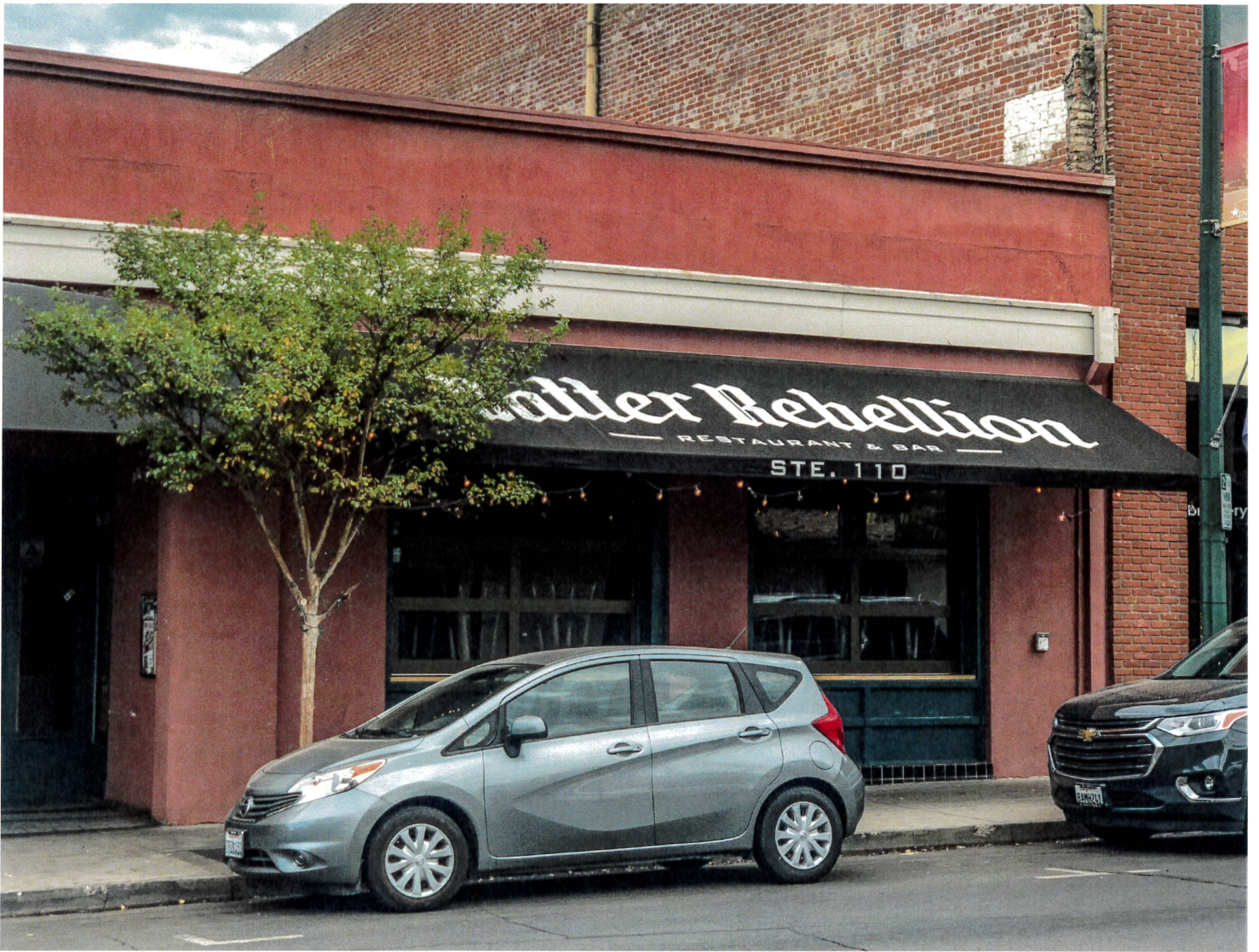
SOUTHEAST CORNER ELEVATION (CITRUS AVE. SIDE)
