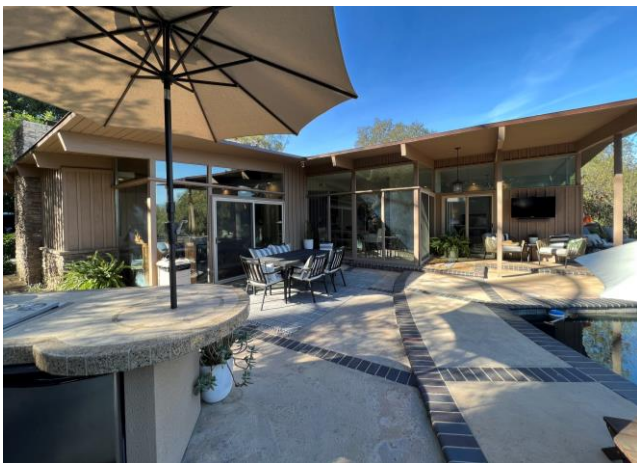
North and east façades, Baker Residence, facing southwest.
