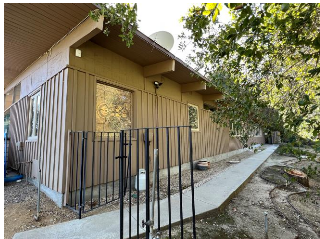
North and West Façades, Baker Residence, facing southeast.
