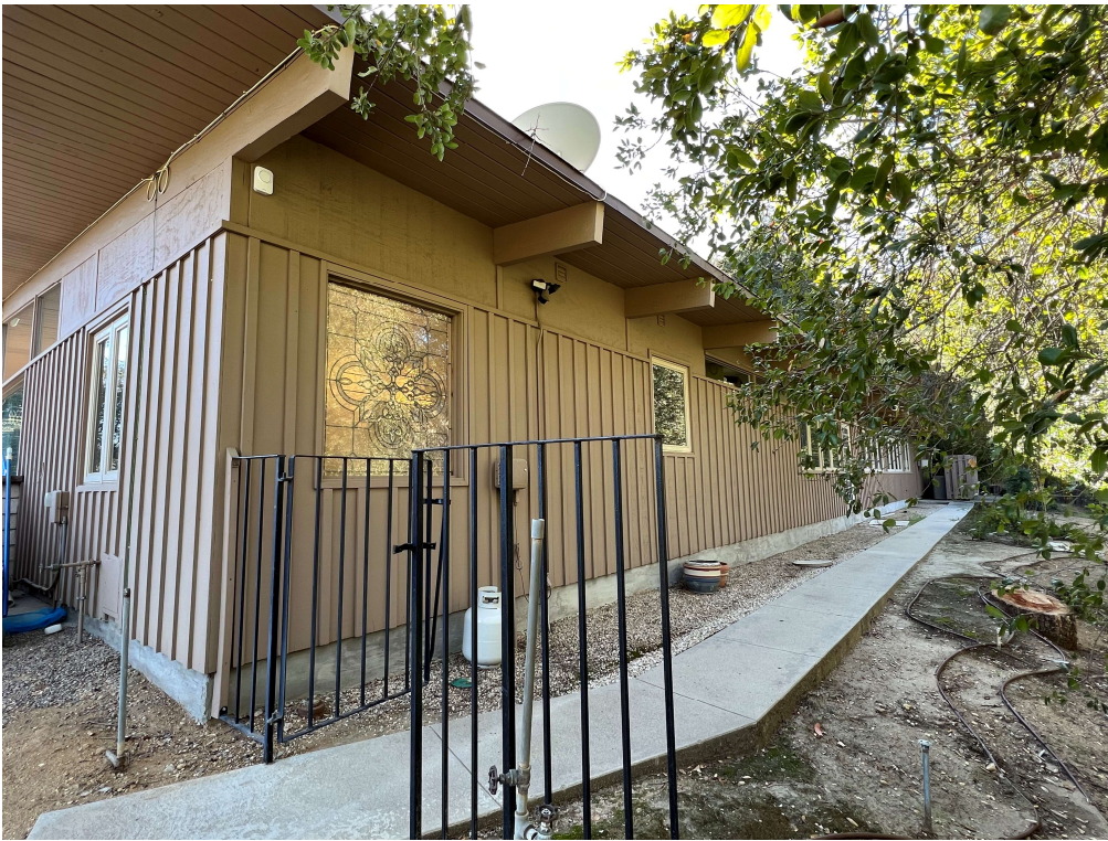
North and West Façades, Baker Residence, facing southeast.
