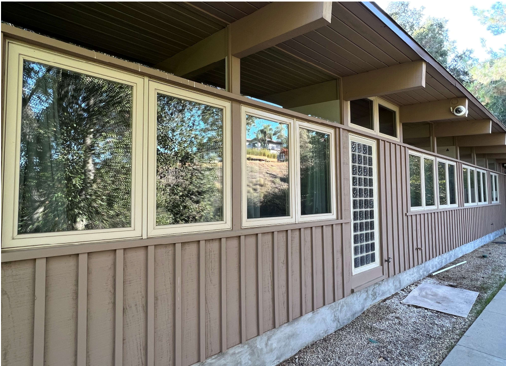
West façade, Baker Residence, facing southeast.
