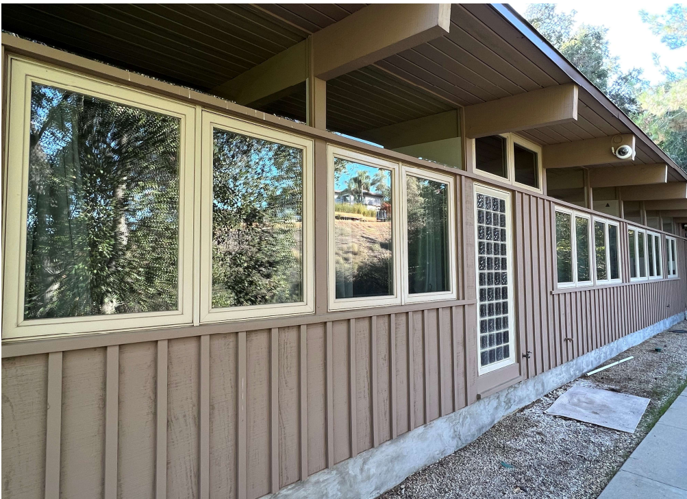
West façade, Baker Residence, facing southeast.
