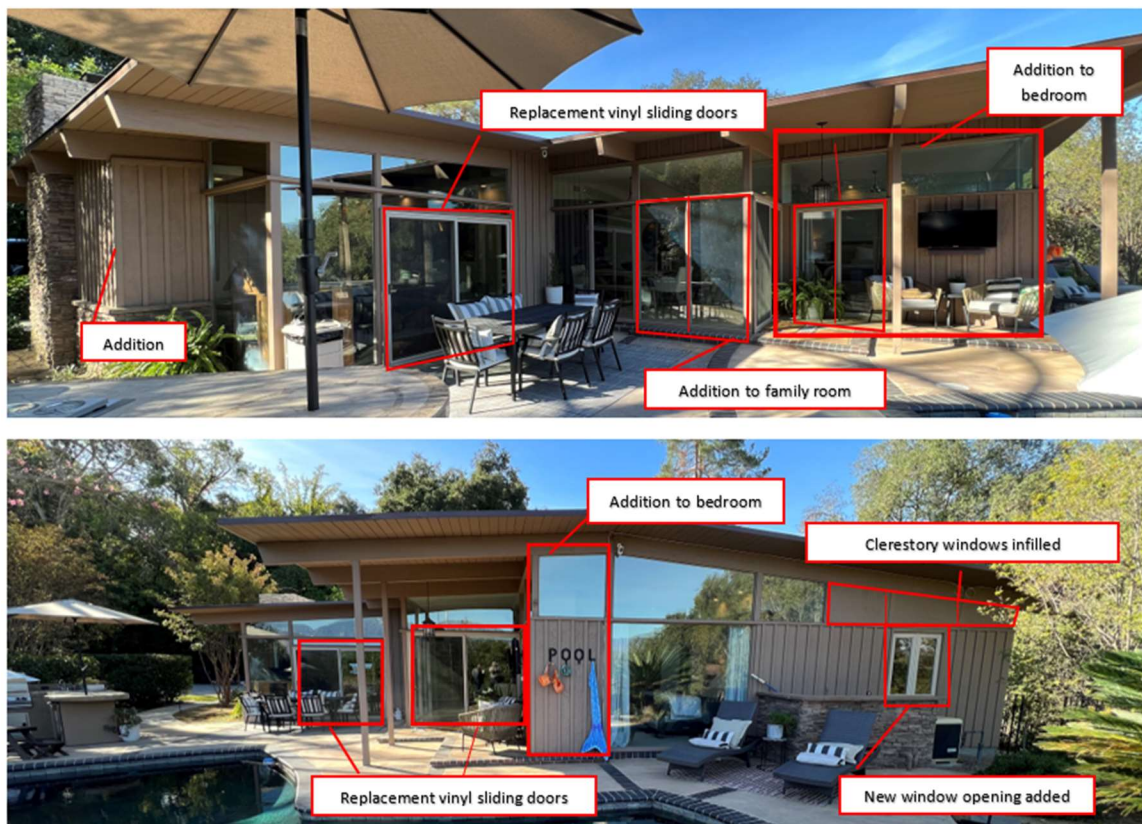
Photographs showing window/door replacement and additions/expansions in red. Source: HRG.
