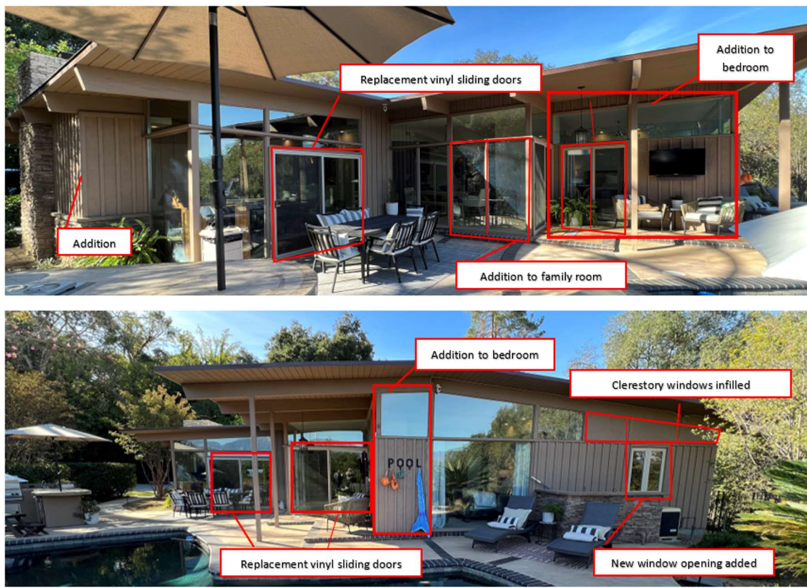
Photographs showing window/door replacement and additions/expansions in red. Source: HRG.
