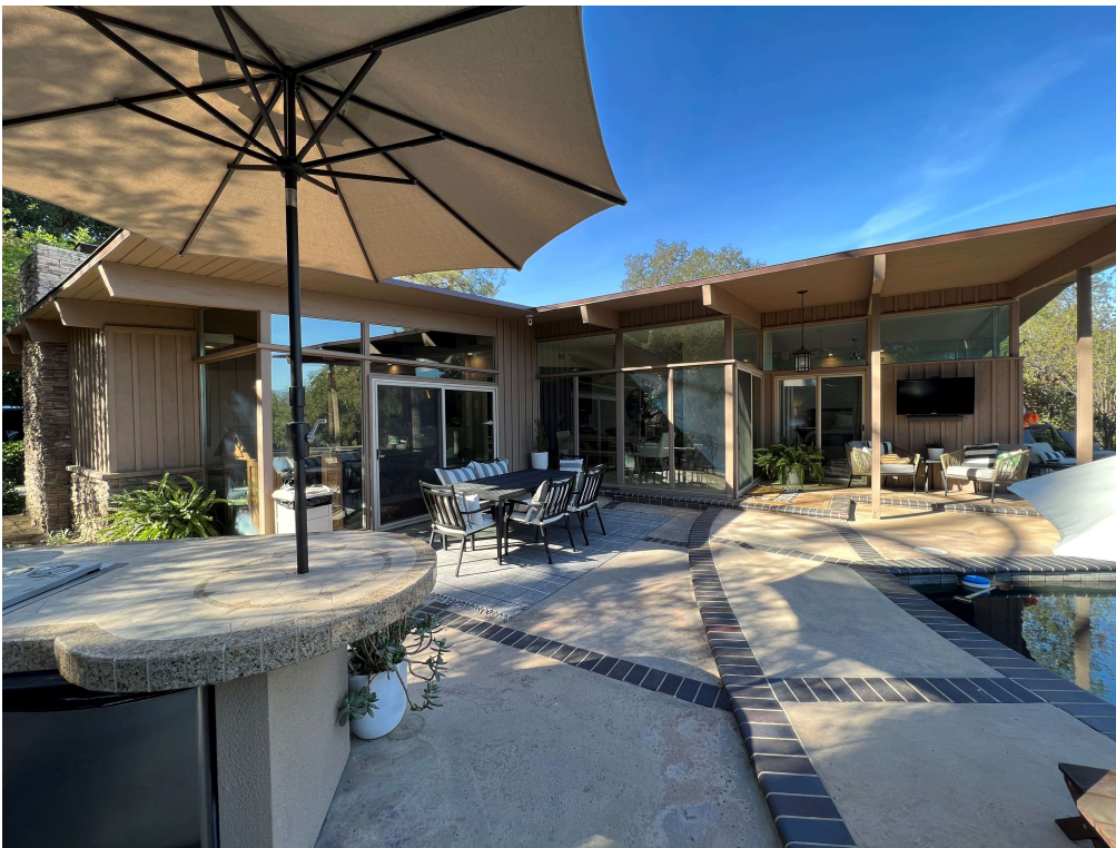
North and East Façades, Baker Residence, facing southwest.
