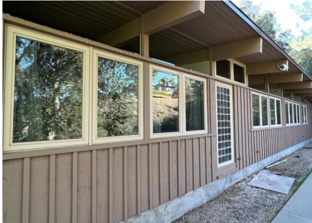
West façade, Baker Residence, facing southeast.
