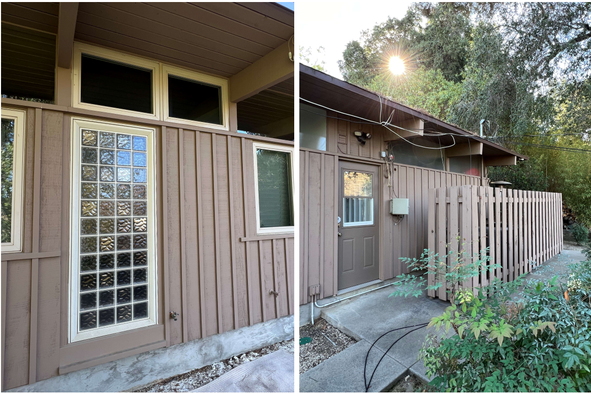
Detail of Doors, West façade, Baker Residence, facing east.
