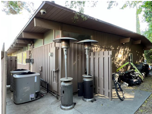
West and east façades, Baker Residence, facing northwest.
