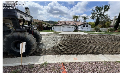
Cement treatment of subgrade on Buckingham Dr
