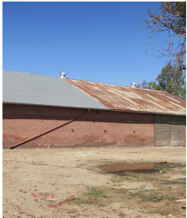
Metal roof on a ca. 1906 warehouse building.
