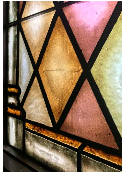
Cracked glazing in a stained glass window.
