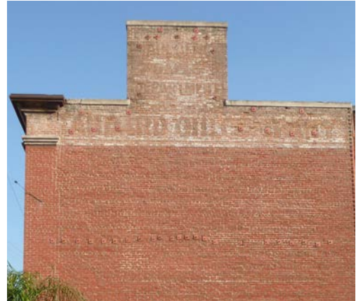
Restore a missing historic sign, such as this painted sign, based on historic documentation.
