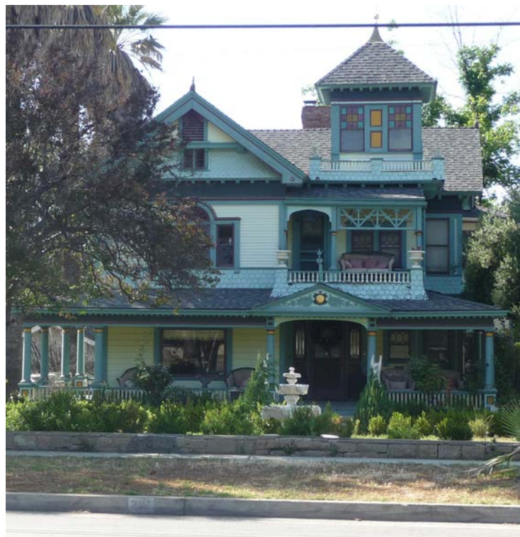
A Queen Anne style house with multiple types of wood cladding and decorative trim.
