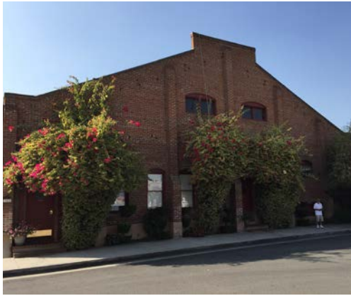
Brick pilasters provide some articulation to this industrial building.
