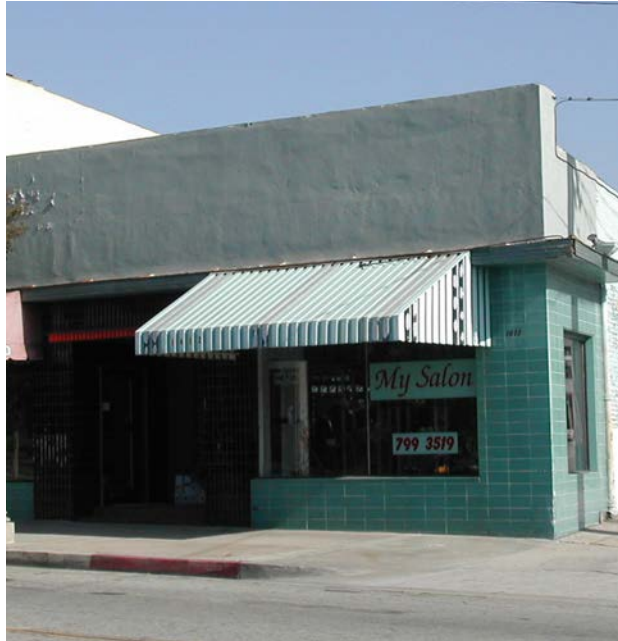
Restore a historic canopy that has been removed or changed to an incompatible style.
