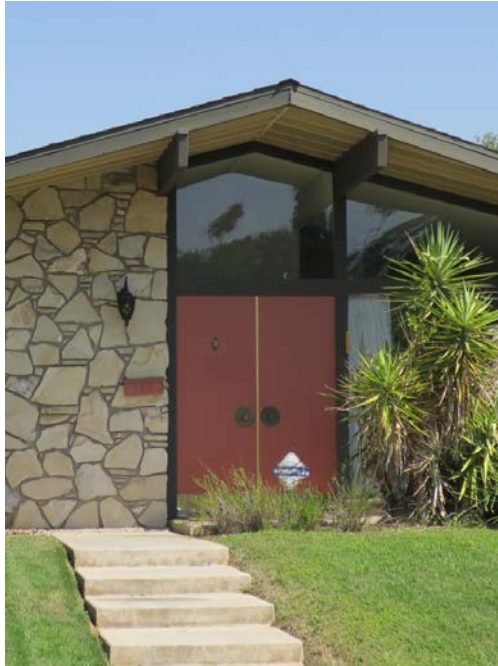
Paired wood slab doors are an important architectural feature of this Contemporary Ranch style house.
