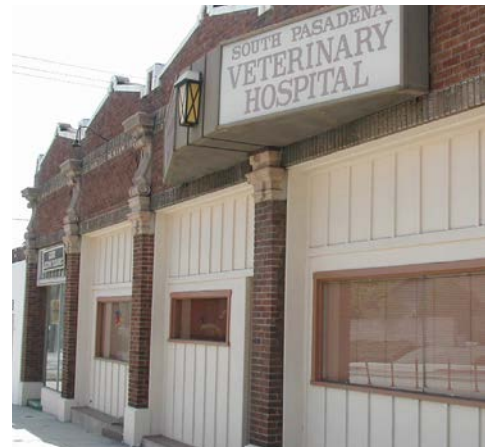
Restore historic architectural features that are missing or are covered up.
