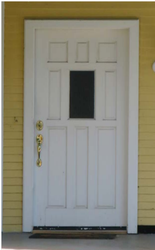
Maintenance, such as repainting and adding new glazing putty, will prolong the life of a historic door.
