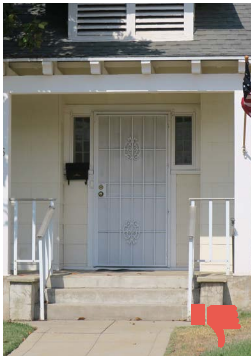
Avoid installing a metal security door that obscures the original historic door from view.
