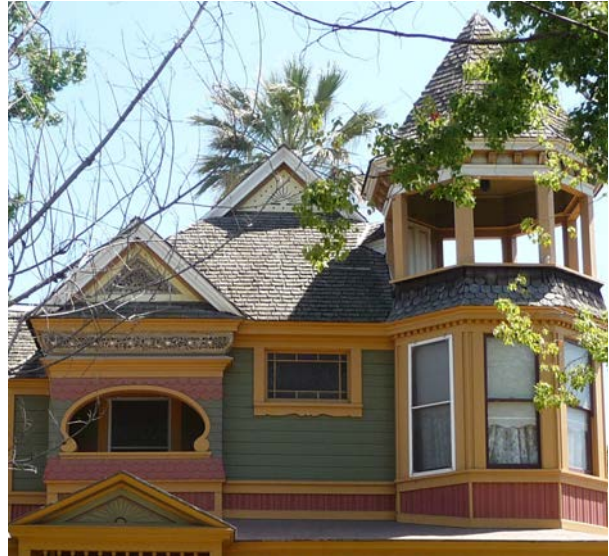
Wood shingle roofing on a Redlands Queen Anne house.
