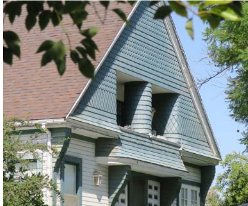
Wood shingle wall cladding.
