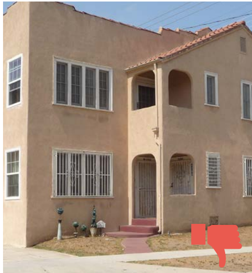
Avoid the use of security bars and doors that obscure historic fenestration.
