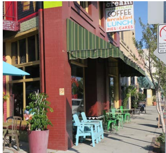
Example of a traditional, triangular-shaped awning, typical of a historic building.
