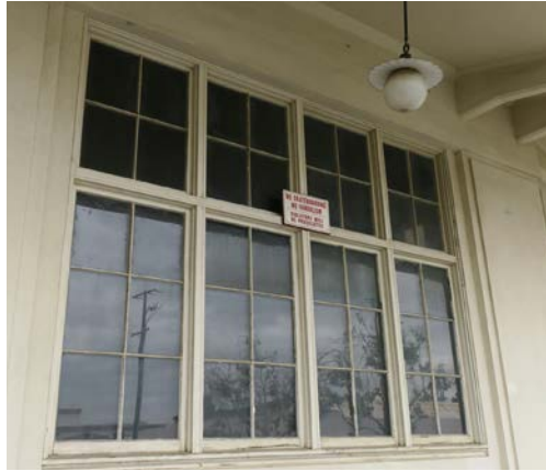
Grouped multi-light wood windows at the Santa Fe Depot.
