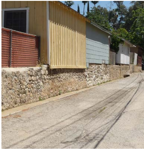
Arroyo stone foundations are an important architectural feature of many historic houses in Redlands and should be preserved.
