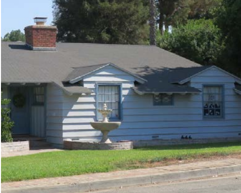
An example of the types of windows and doors that are appropriate for Redlands' postwar neighborhoods.
