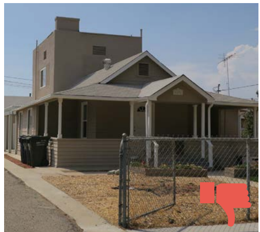
Avoid additions that are not compatible with the scale and style of the building.
