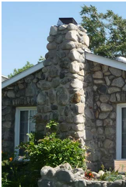
Exterior stone chimney.
