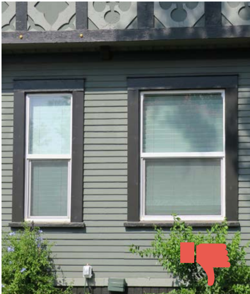
Avoid replacing windows with stock items that are incompatible with the historic materials or colors of the building.
