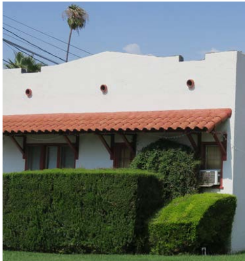
The clay tile awning on this house is an important historic accessory feature that should be preserved.
