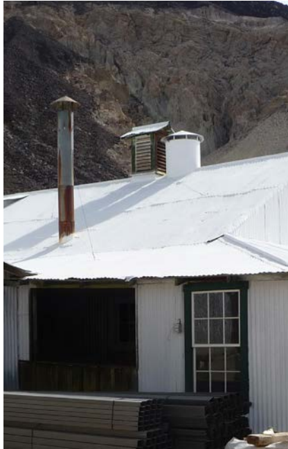
Roof with multiple penetrations and flues.
