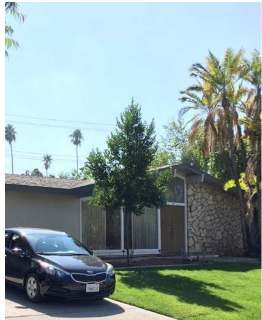
An example of stucco cladding and stone accent cladding, typical of houses in Redlands' postwar neighborhoods.
