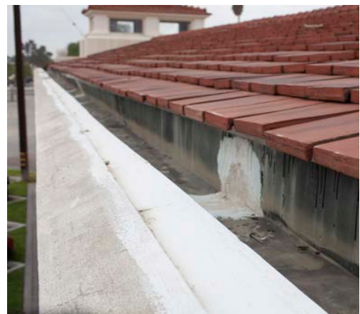
Integral gutter at Santa Fe Depot.
