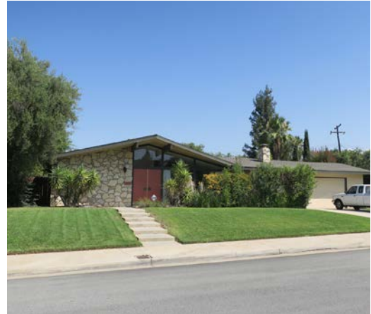
Postwar developer-built houses are typically one story with horizontal massing.
