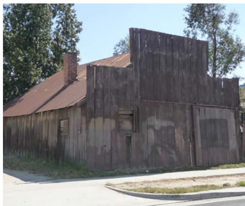
Vertical board cladding on a ca. 1908 blacksmith shop.
