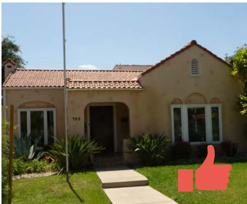
An example of a minimally visible, appropriate roof addition at the rear of a building.
