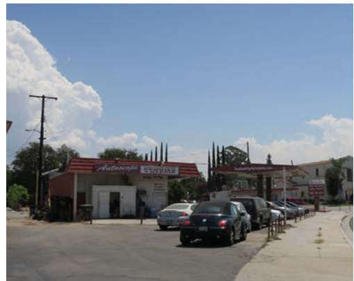
Parking at this auto-oriented building is prominently featured at the front of the building.
