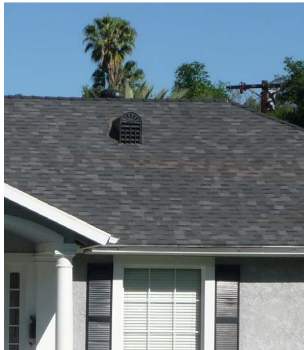
Composition shingle roofing.
