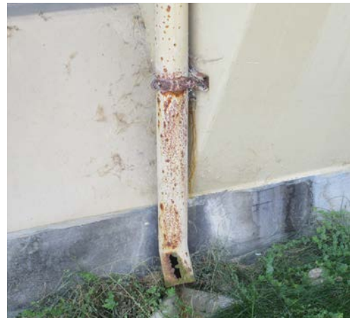
Corroded downspout.
