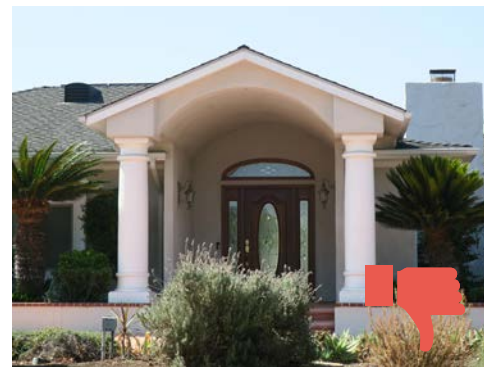
Avoid adding new features that are not appropriate to the architectural style of a building, such as classical columns on a Ranch style house.
