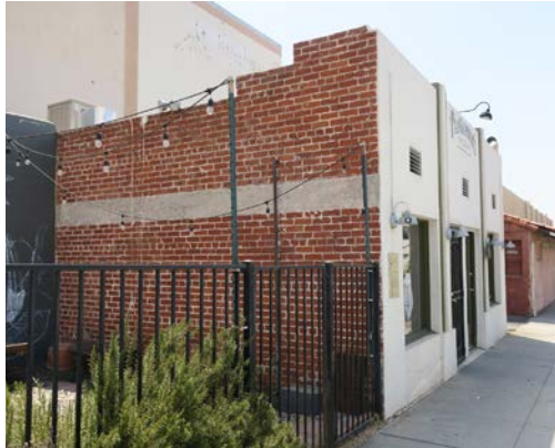
A metal fence defines the side yard of this commercial property.
