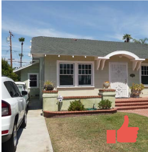
An example of an appropriate addition to a historic building. The addition is located on the side façade, set back from the front of the building; it is smaller in footprint and subordinate to the main building, and its roofline has a similar pitch as the historic roof pitch.
