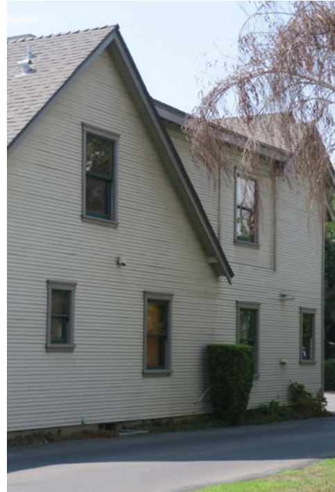
A historic rear addition.
