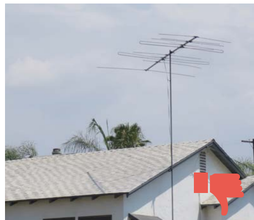
Avoid installing utility features, such as this antenna, at the front of a building.
