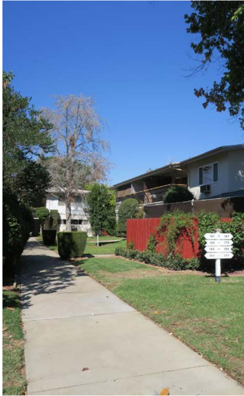
Pedestrian access to this garden apartment complex is provided via a paved walkway.
