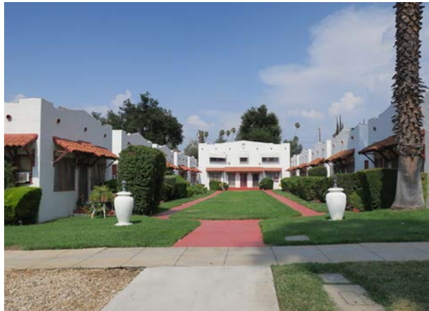
A multi-family residential development in southwest Redlands.
