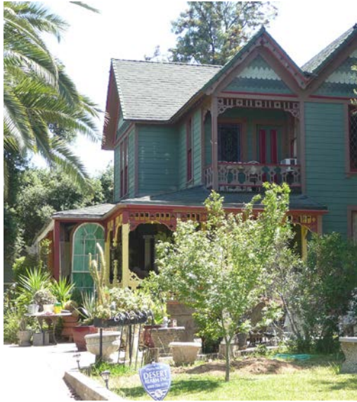
Decorative gingerbread details and multi-colored shingles are defining features of Queen Anne and Stick architecture that should be preserved.
