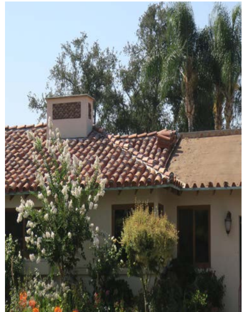
New roof tiles or shingles should match the material, size, profile, and color of the historic roof as closely as possible.
