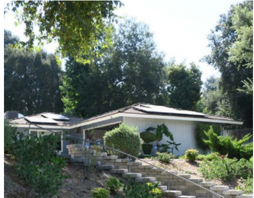
A low-pitched roof, typical of postwar architecture.
