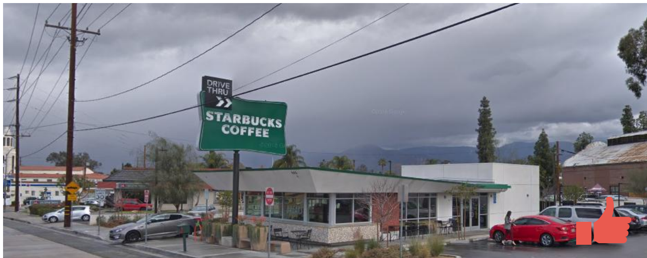
A simple one-story rear addition is compatible with the scale and design of this historic drive-thru restaurant. (Image, Google, 2018)
