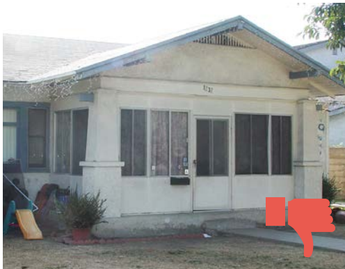
Avoid enclosing a historic porch at the primary entrance to the building.
