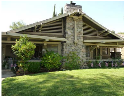
Wood roof details on a Craftsman duplex.
