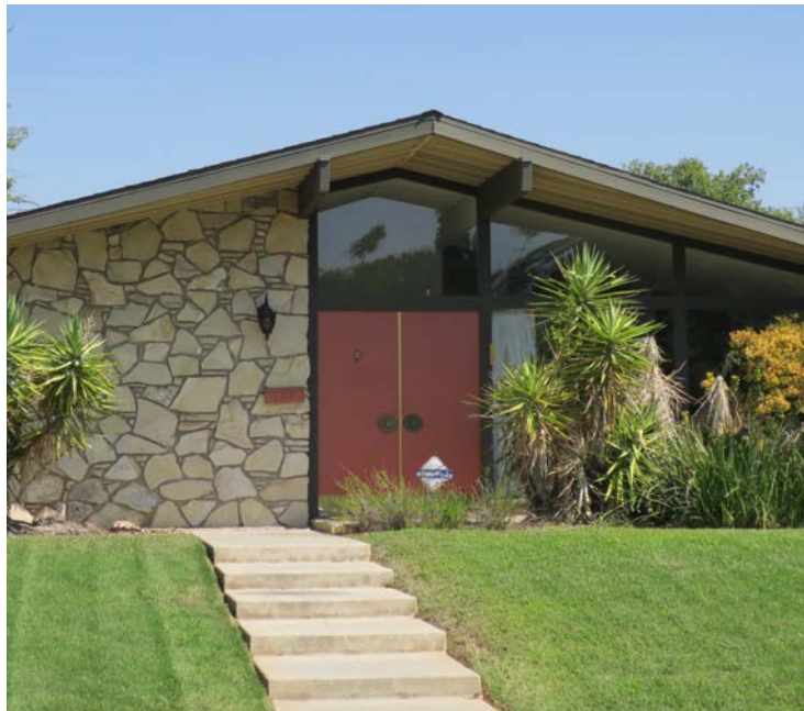
The tall wood doors and clerestory windows on this Contemporary Ranch house are integral to its character.
