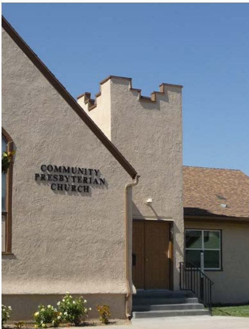
Textured stucco on a Redlands church.
