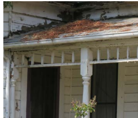
Remove debris from roofs and gutters.
